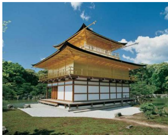
Obrázok 4: Kinkaku-ji (Temple of the Golden Pavilion) Zdroj: YOUNG, M., YOUNG, D.: The Art of Japanese Architecture . North Clarendon : Tuttle Publishing, 2007. s. 84-86.
