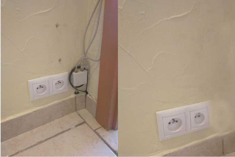
Figure 3: Installation of engineering networks before and after treatment
