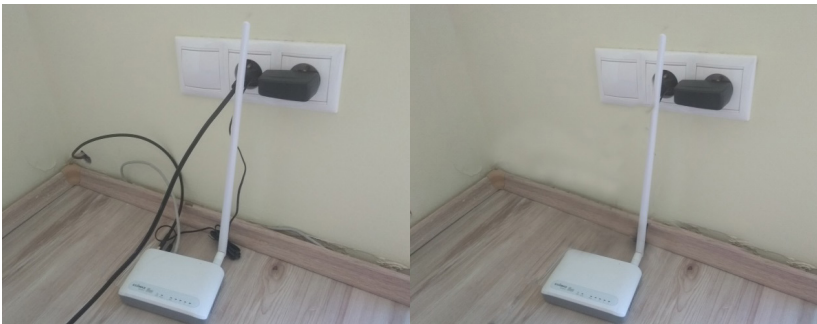
Figure 2: Installation of computer network wiring for and after retouching
