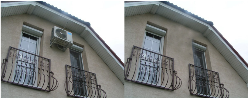
Figure 4: Installing the split outdoor air conditioner with and without installation
